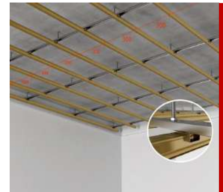
Install the triangular profile
